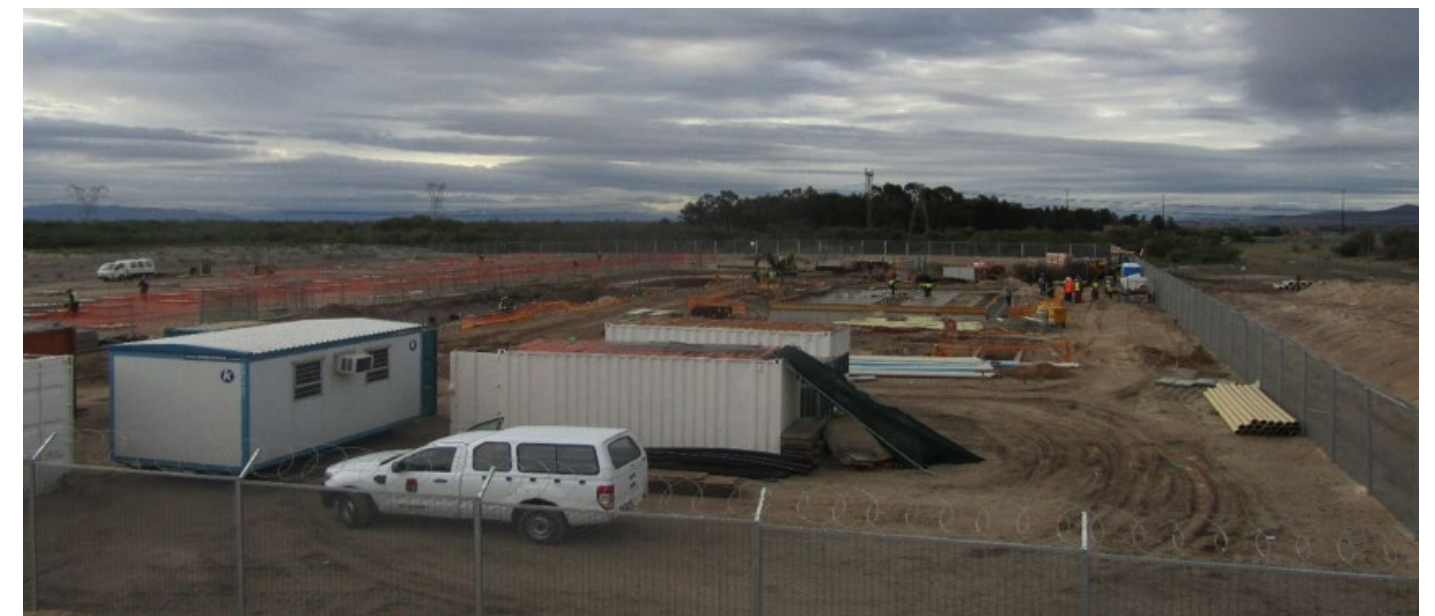
- Construction work in progress at the new sub-station in Atlantis
