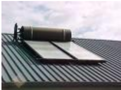
Retro-fit of Solar Water Heating
