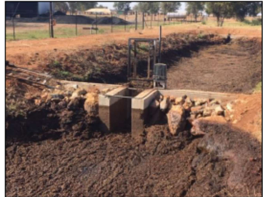
Figure 5.7: Settling dams with moving screen filter at facility 3013.5 (Angle 2)
