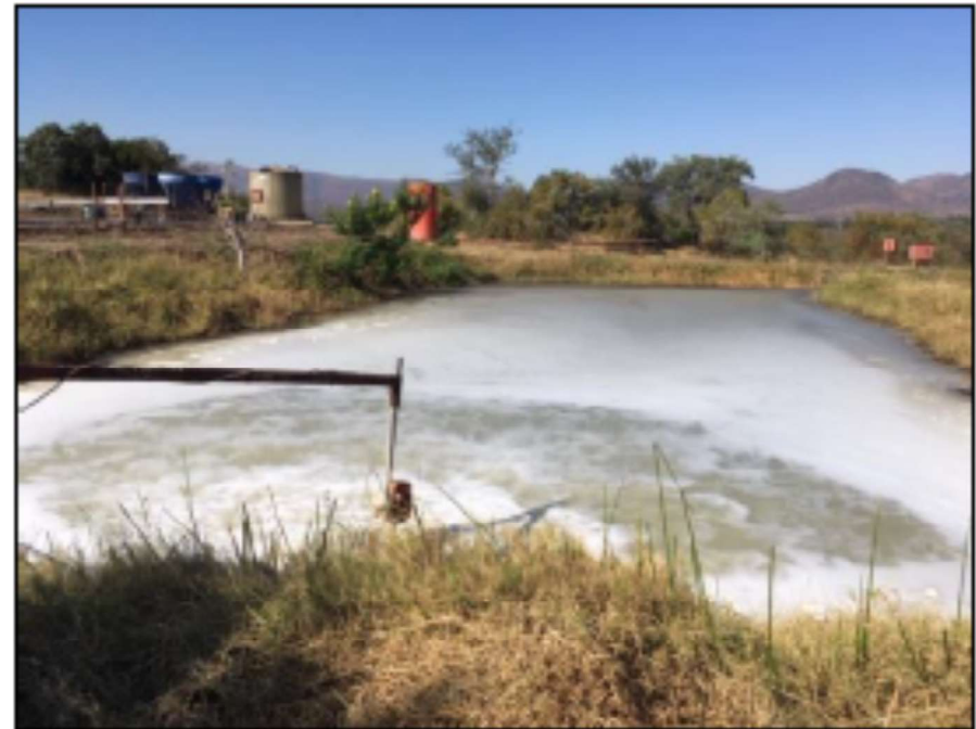
Figure 5.5: Aerobic lagoons (with aerator) used at facility 3103.2
