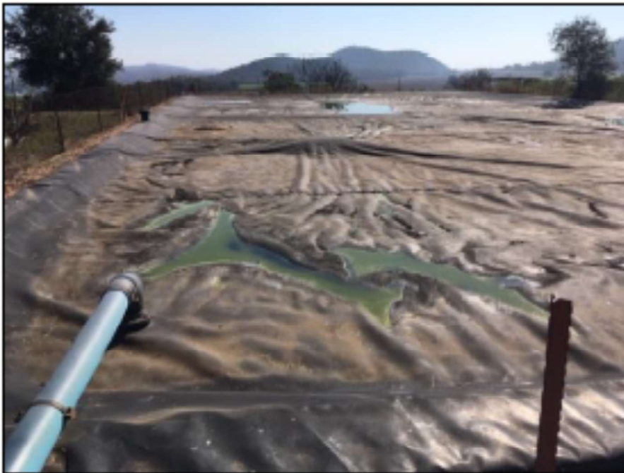
Figure 5.4: Anaerobic lagoons used at facility 3103.2
