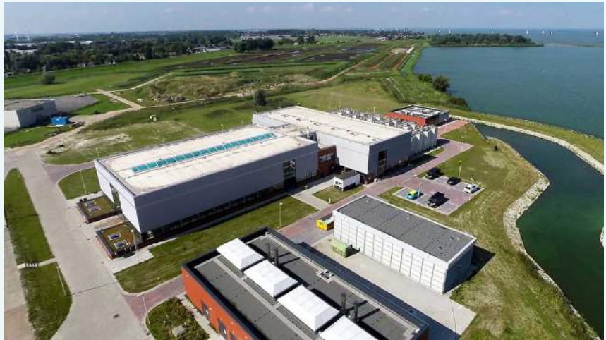
Andijk III water treatment plant produces 120 million liters per day from surface water, using suspended ion exchange (SIX®) and ceramic membranes (CeraMac®)
