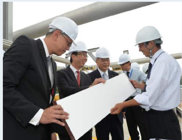
Site tour of the UASB-Ceramic MBR plant
