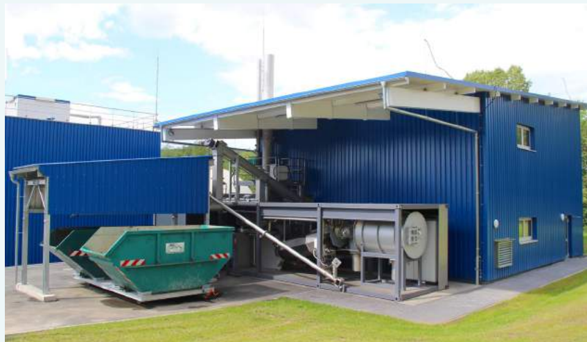
The Pyreg plant at Linz-Unkel in Germany
