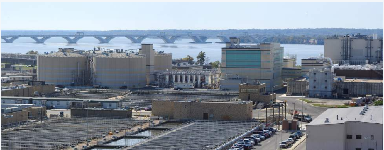
DC Water Biosolids plant at the Potomac River
