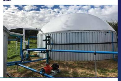
WISP worked with Global Energy to identify Rennie Farms as a suitable location to invest R 1 200 000 into the development of an anaerobic digestion plant. The plant successfully produced biogas from a daily supply of 1.5 tonnes of organic vegetable waste from Rennie Farms.
